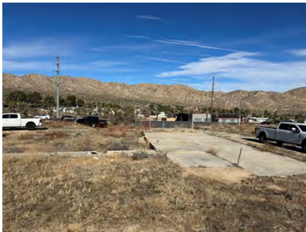
Figure 5-2. Concrete foundation remnant in western portion of APE, facing north.
